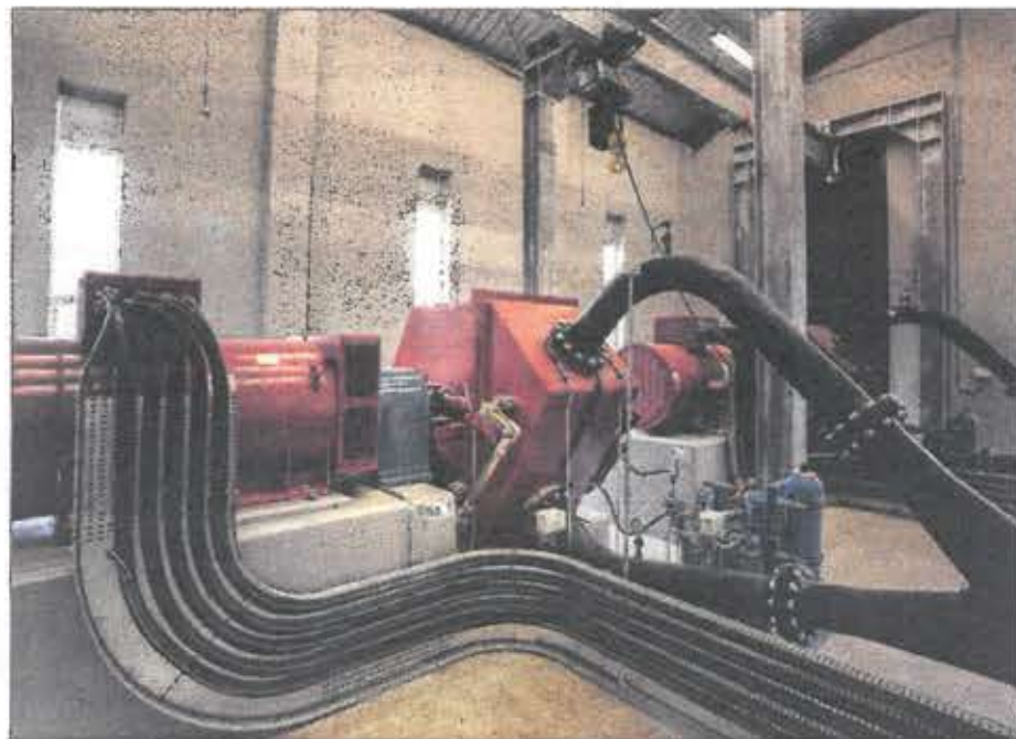
■ The massive Ossberger turbine generator sets, left, crouch like athletes at the start line, waiting for the pipeline from the weir in the mountains far above L'Ormarins Wine Estate, to deliver the at least 35 litre per second they need, to come to life and start to generate green energy.
